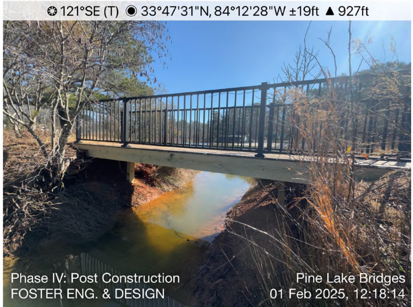
IMG_8513 – Second pedestrian bridge
