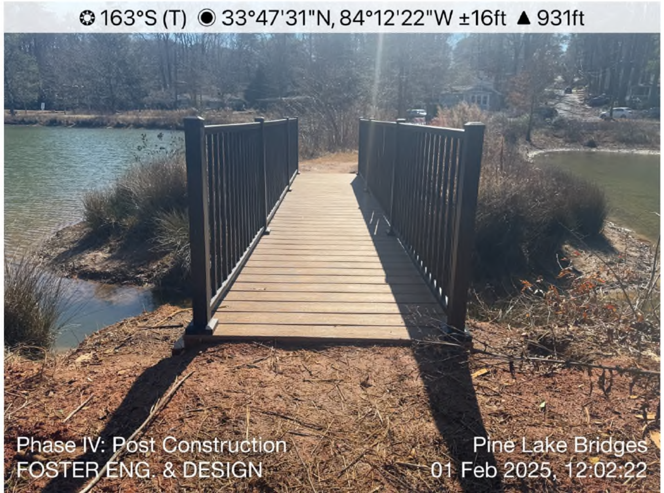
IMG_8483 – First pedestrian bridge
